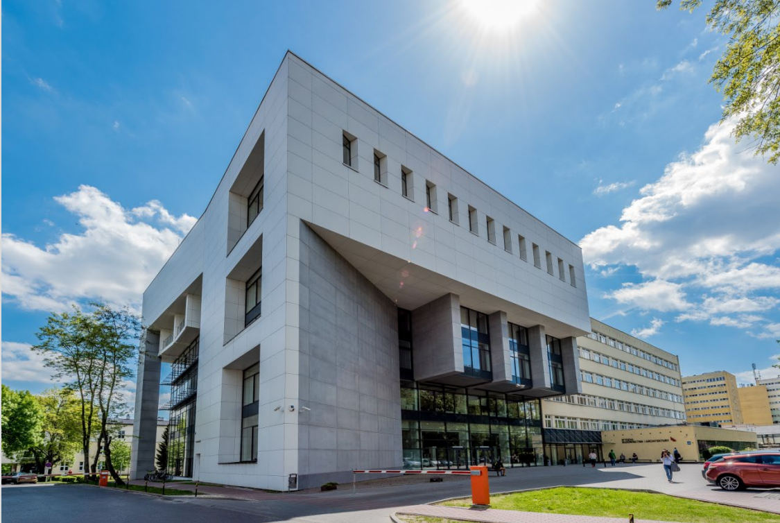
Faculty of Civil Engineering and Architecture
