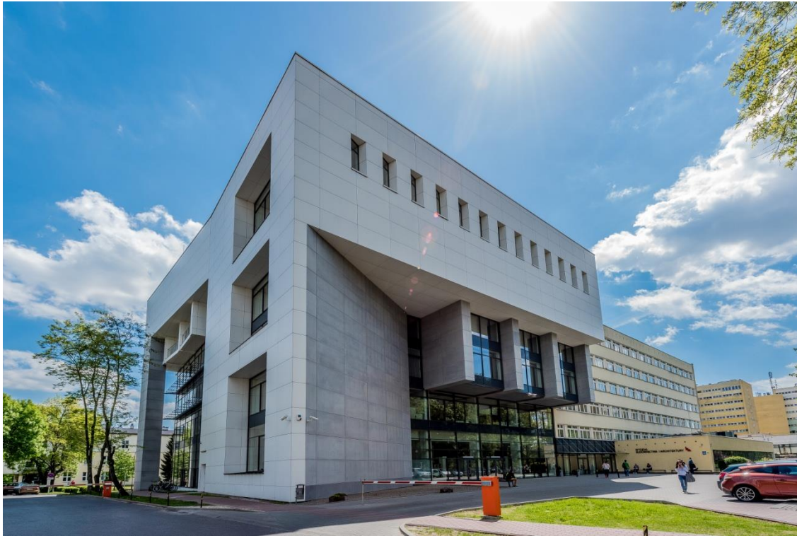
Faculty of Civil Engineering and Architecture
