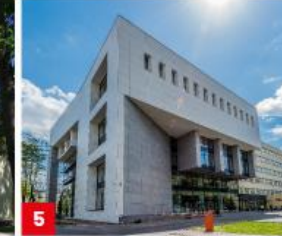
5 FACULTY OF CIVIL ENGINEERING AND ARCHITECTURE
