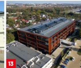
13 CENTER FOR INNOVATION AND ADVANCED TECHNOLOGIES
